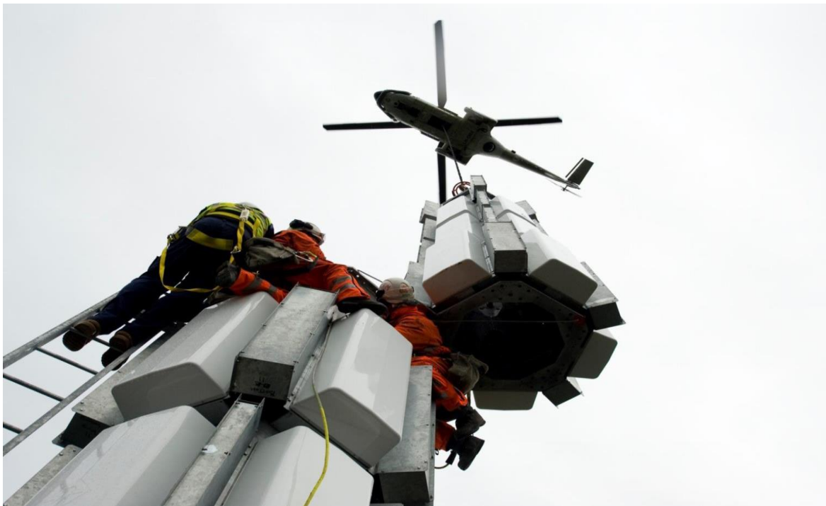
Figure 7 A helicopter being used to install an antenna 10
